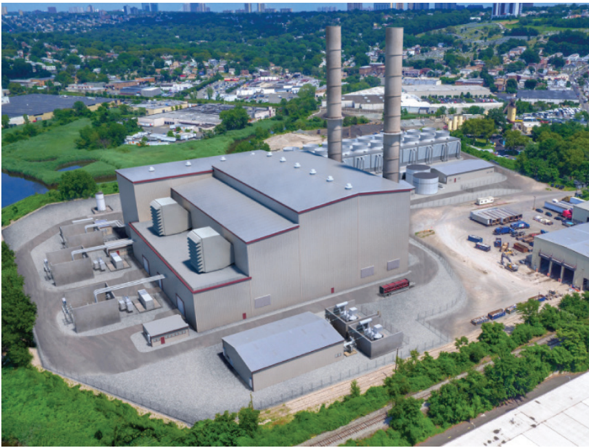
In the event of storm surge and rising sea levels, the proposed NBLG power plant (illustrated here) is at risk of flooding as it lies on the banks of the Hackensack River in North Bergen, NJ. Image source: NBLG
