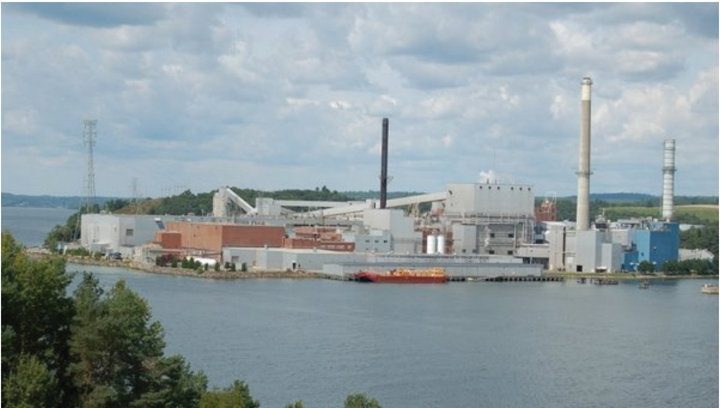
The paper mill in Bucksport that Whole Oceans is renovating to be their aquaculture facility.
