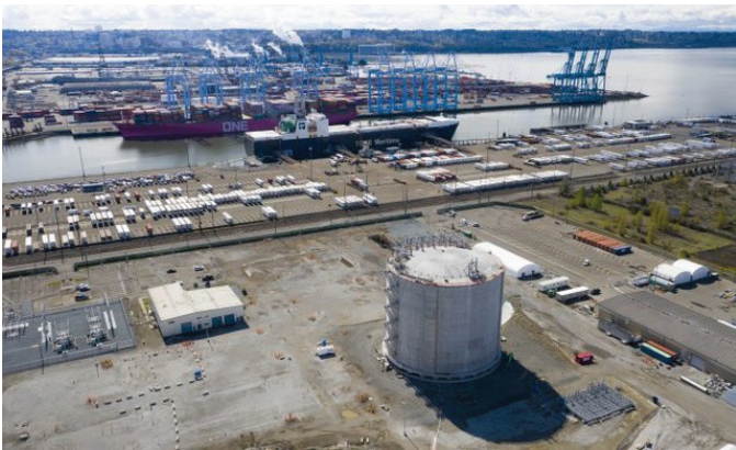
Port of Tacoma LNG plant (Source: Port of Tacoma)
